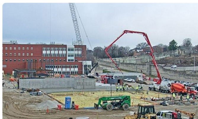
Construction of the new General Headquarters Crime Laboratory.
